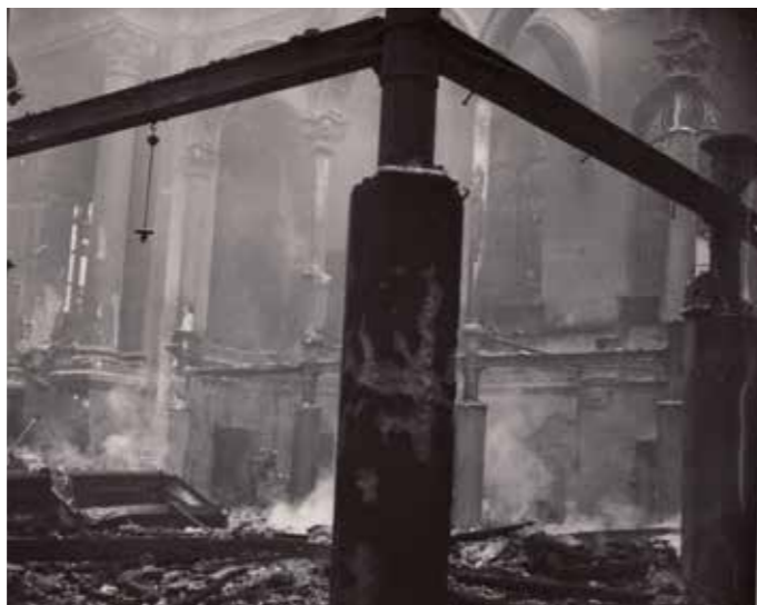
Extinguishing the last fires in the burnt out synagogue. Photograph of Stanislav Maršál. Archives of VHÚ, Prague.
